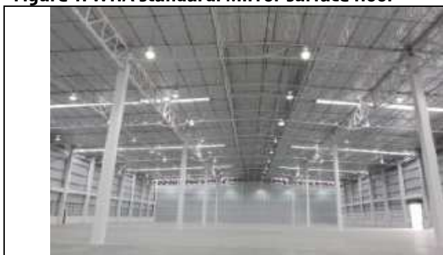
Figure 1: WHA standard: Mirror surface floor
