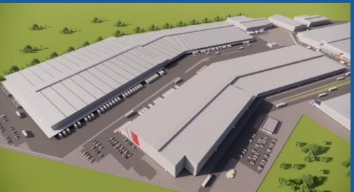
Retail and Construction Materials 38,000 sqm
